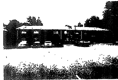
BUILDING 19 (CAROLINA COVE GARDEN UNITS) FRONT
